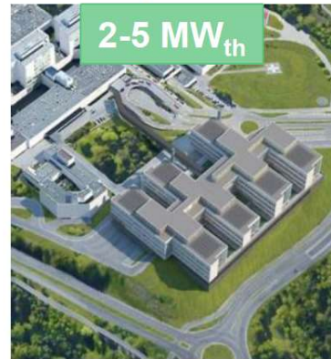
Recovering waste heat from Espoo hospital
